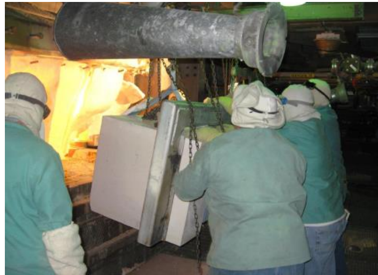
New mantle block being installed
